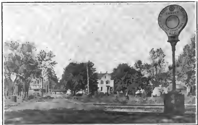
How the Lehigh Valley Railroad proposes to protect dangerous crossings
